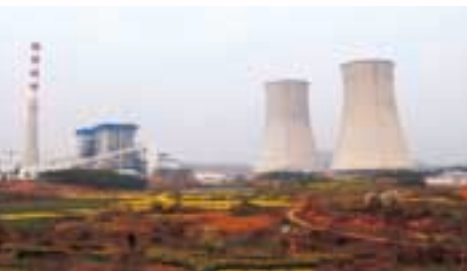
Dabieshan Power Plant
