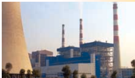
Pingwei Power Plant II
