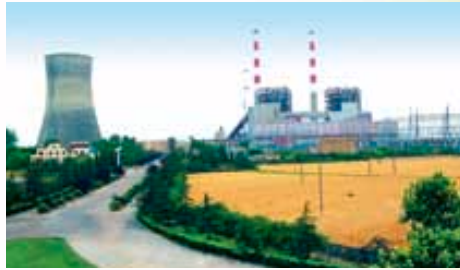
Pingwei Power Plant
