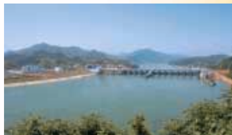
Wu Ling Hydro Power
