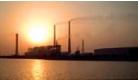
Changshu Power Plant
