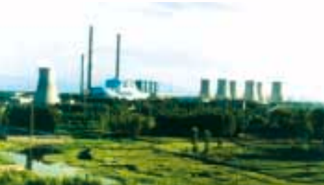
Shentou I Power Plant
