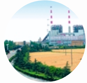
Pingwei Power Plant
