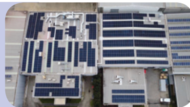
In September 2021, the solar panel system was implemented in Ausnutria's operation building in Australia.
