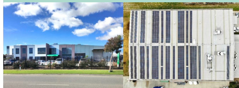
Dairy factory in Australia
